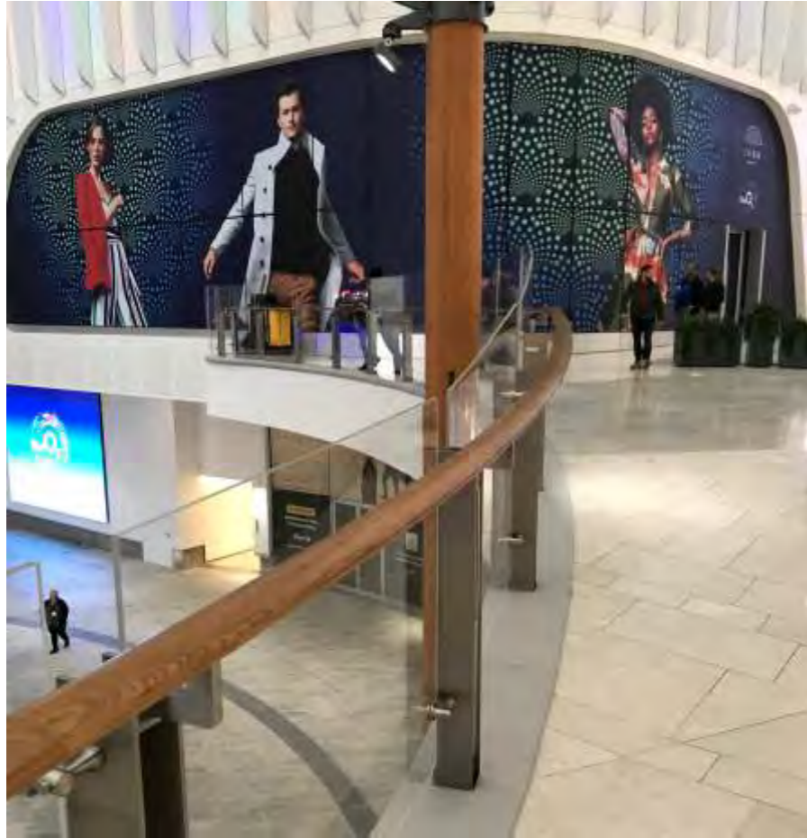
Above photo: Glass and stainless steel balustrade project at the Icon Outlet, O2 Arena.
